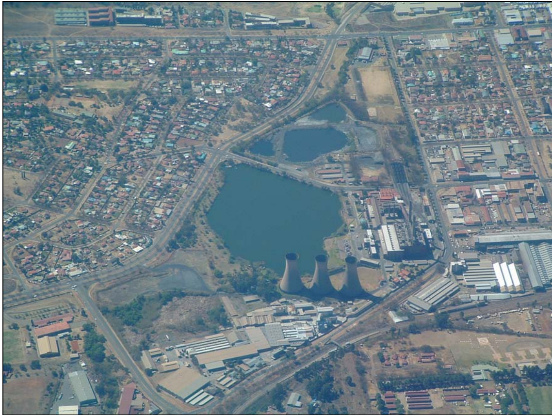
Figure 6: Pretoria West Power Station in the Pretoria West Industrial Area
